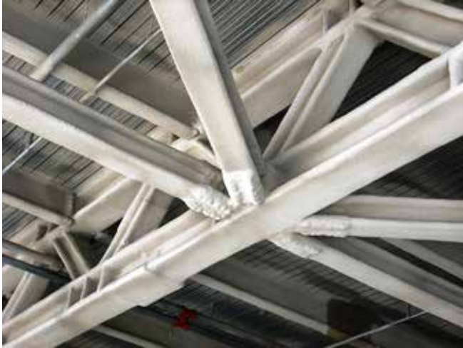
Truss & Tie Beam Connection
